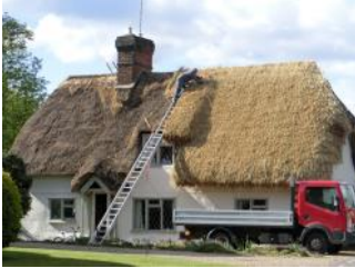
Rickling Green work in progress
